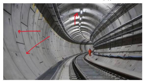
(Smooth panels after TBM method)
