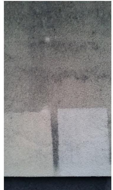
*Photo of the efficiency of functional coating FN<sup>®</sup> 1 on the facade for 7 years*
